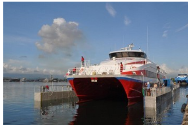
Figure 37 : Dock flottant 45 m (source HT2)
